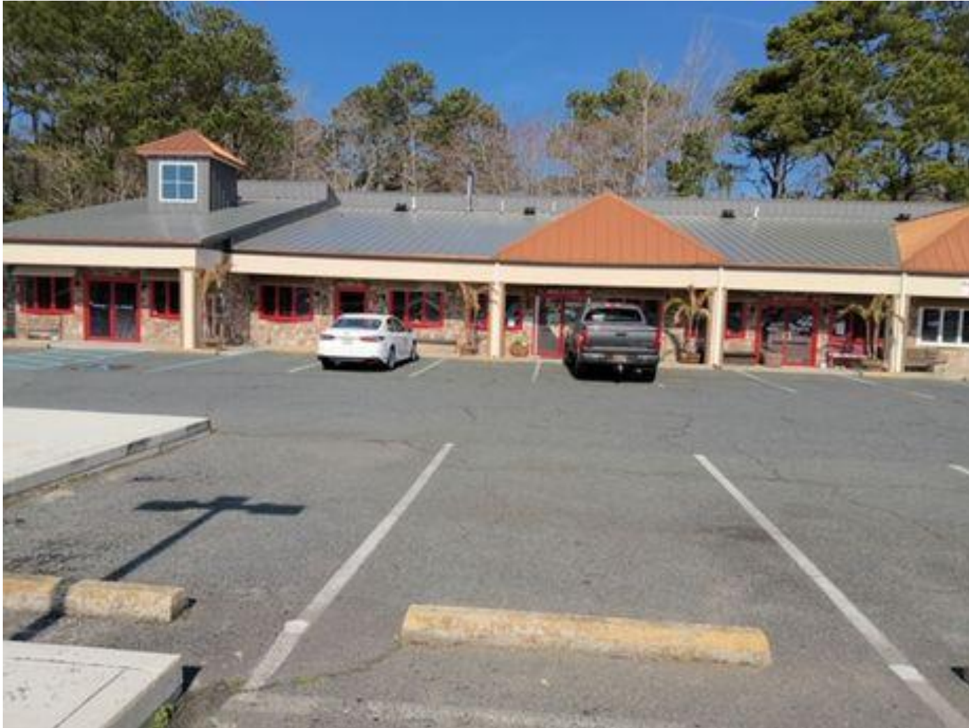
Overall Front of Licensed Premises from Route 50
