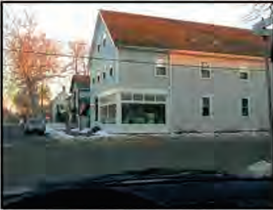
Adaptive reuse suits in-town commercial development
