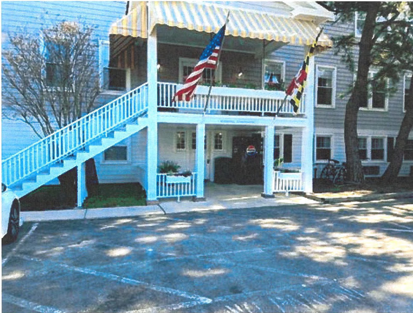
Main entrance to Atlantic Hotel from parking lot.
