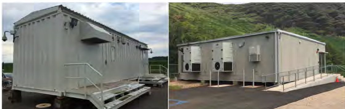
Figure 2 – PFE building examples
