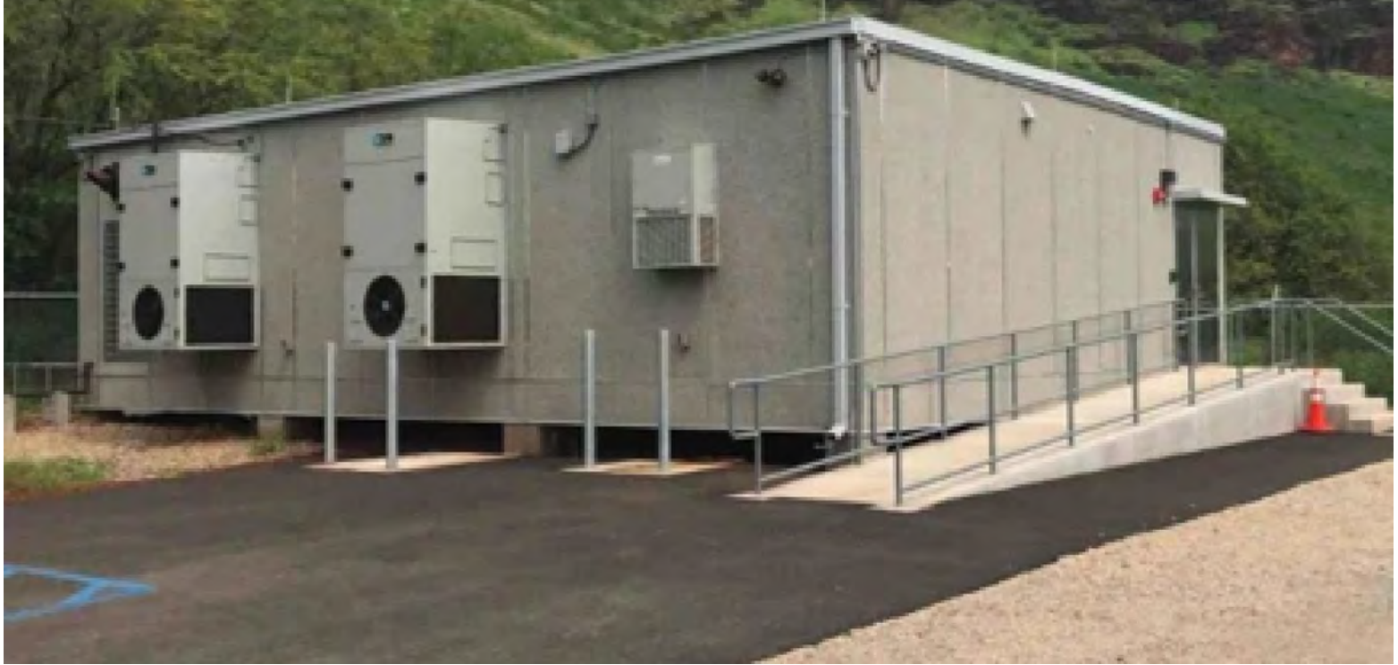
Figure 3 – PFE building examples
